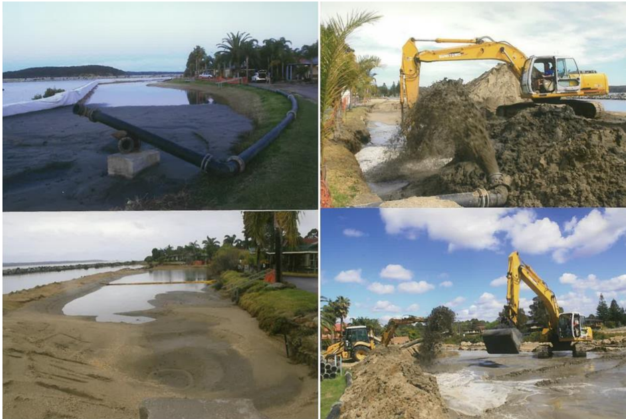
Figure 50: View of land reclamation works undertaken at the site, showing pumping of clean sand
