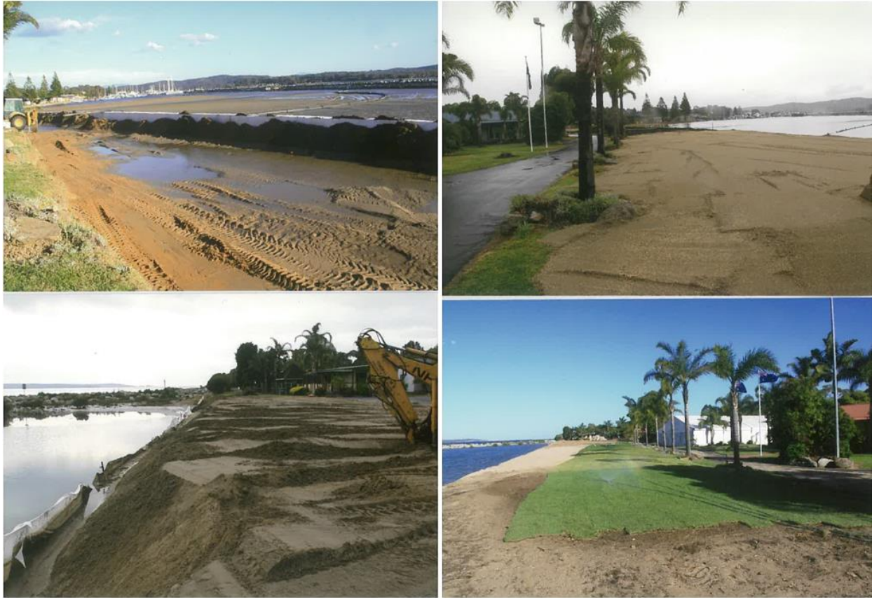
Figure 51: View of land reclamation works undertaken at the site, showing pumping of clean sand
